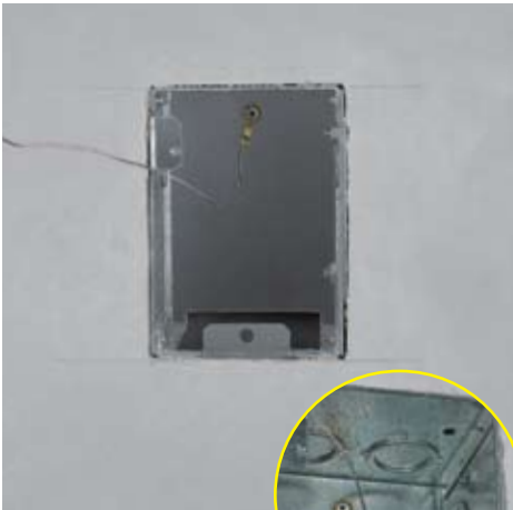
XEM box (provided) replaces standard junction box for rough-in installation. Multiple options for wiring access available through knockouts (inset). Notches in mounting bracket indicate correct placement for 1/2", 5/8" and 1" wallboard.
